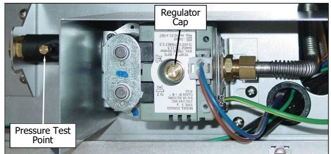
**NOTE:** The Pressure Test Point is located behind the front service panel beneath the oven door.
